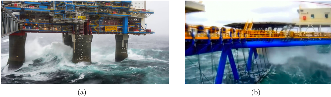
Figure 2: Extreme waves impact on an offshore O&G platform Normannsen (2021) and a bottom-supported fish farm through the live monitoring system.
