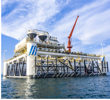
(c) Bottom-supported smart fish farm Jinghai No. 1
